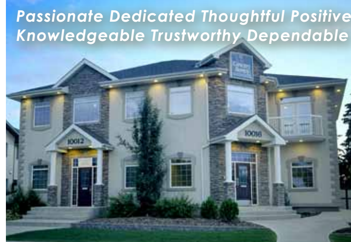
Concept® Homes Main Office building
