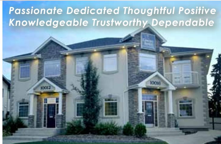
Concept® Homes Main Office building
